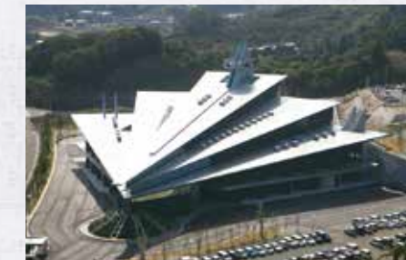
Uzushio Electric Co., Ltd. MIRAI Factory This company is one of the biggest manufacturers of electrical equipment for ships in Imabari. The idea for the design of the factory comes from future ships. It looks like a space ship in sci-fi movies.
