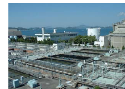
A Distant View of Primary Sedimentation Tank and Sludge Treatment Building
