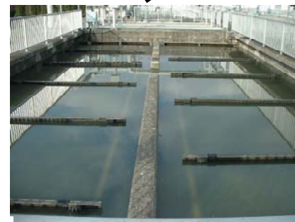
Primary Sedimentation Tank
