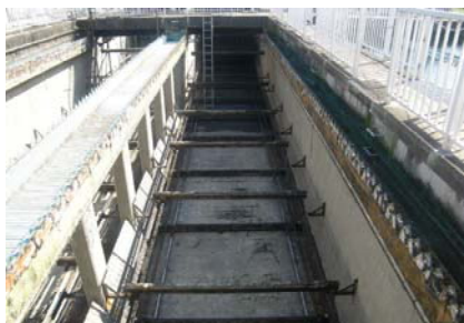
Final Sedimentation Tank (Inner Structure)
