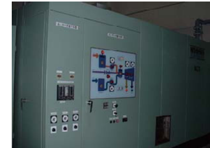
Sludge Treatment Building
